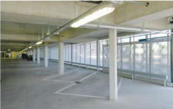
Photo 3: Sous-sol ( Parking ) de Centre Commercial COOP «Le Cârô» (source: https://www.architectes.ch/fr )
