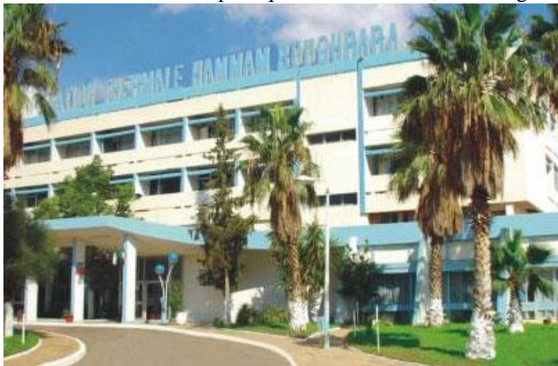
Figure 07 : Station thermal de Hammam Boughrara
