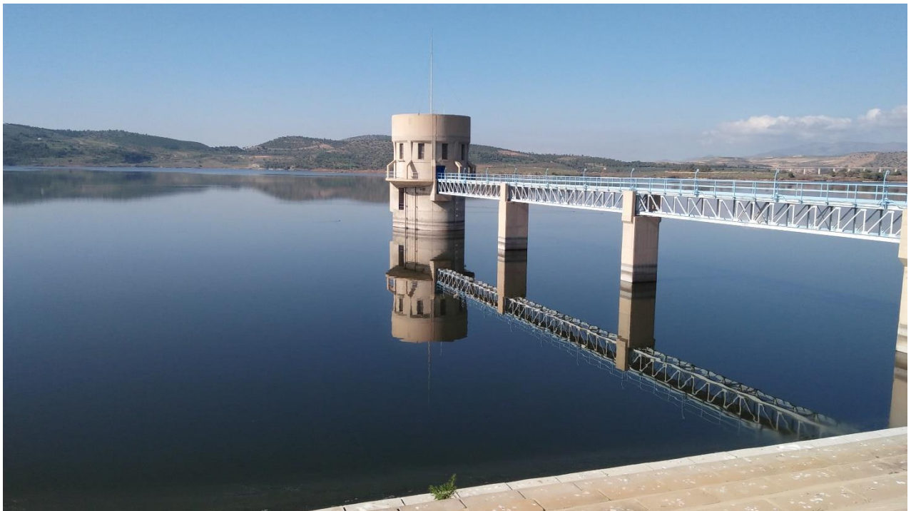
Figure 34: Barrage de Hammam Bouhrara (Chater,2019)
