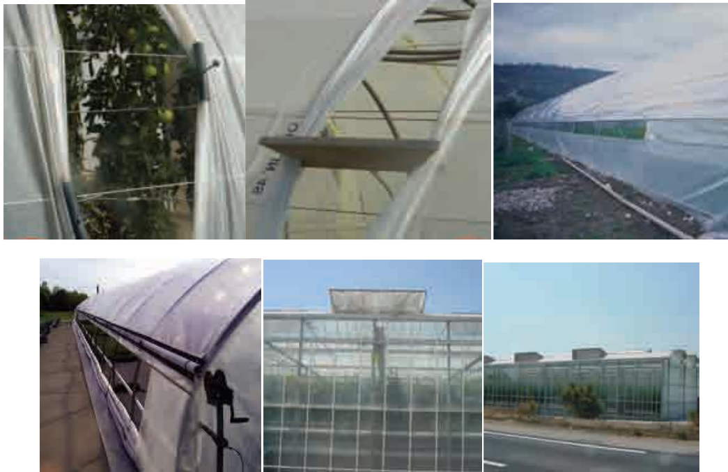
Figure 1.8 Different types of ventilation openings
