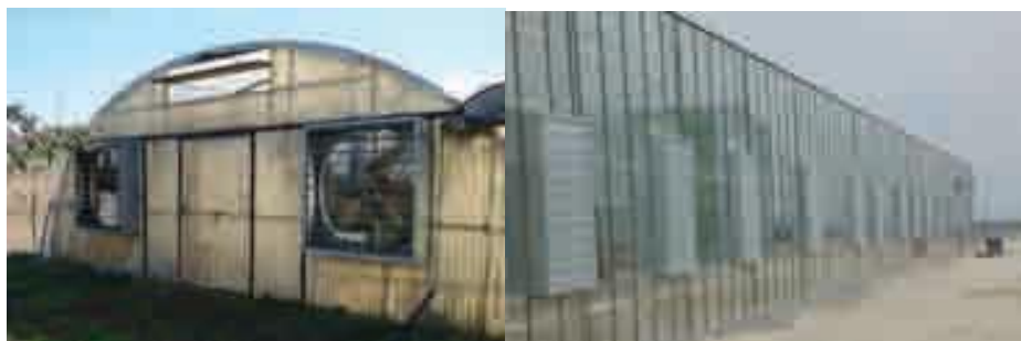
Figure 1.9 Fans for greenhouse forced ventilation
