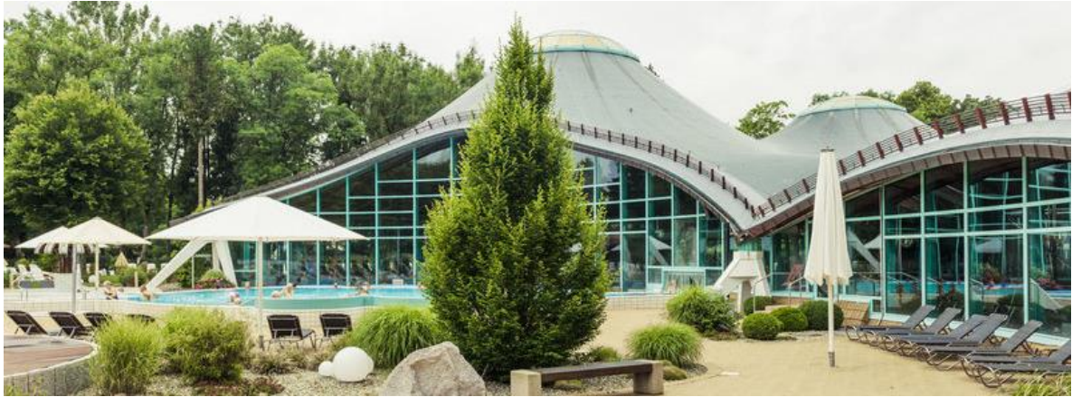
Figure 82: Station thermal 'bad durrheim' a Freiburg, Allemagne.
