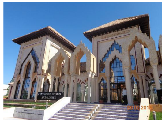
Figure 99: Centre d'étude andalouse.
