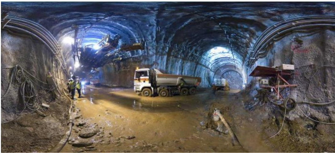
Figure 2.2 Espace souterrain (Bousbia, 2016)
