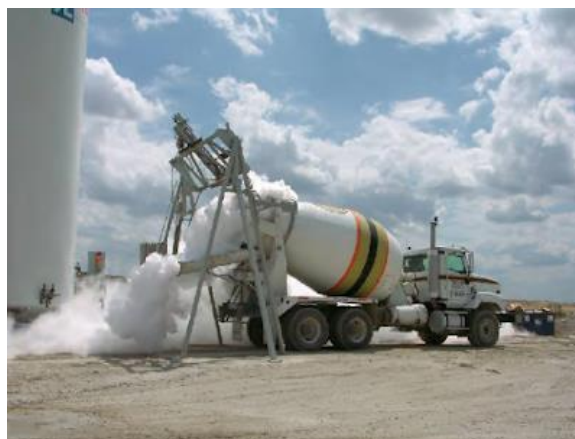
Figure 2-4 Injection of nitrogen directly into a concrete mixer.
