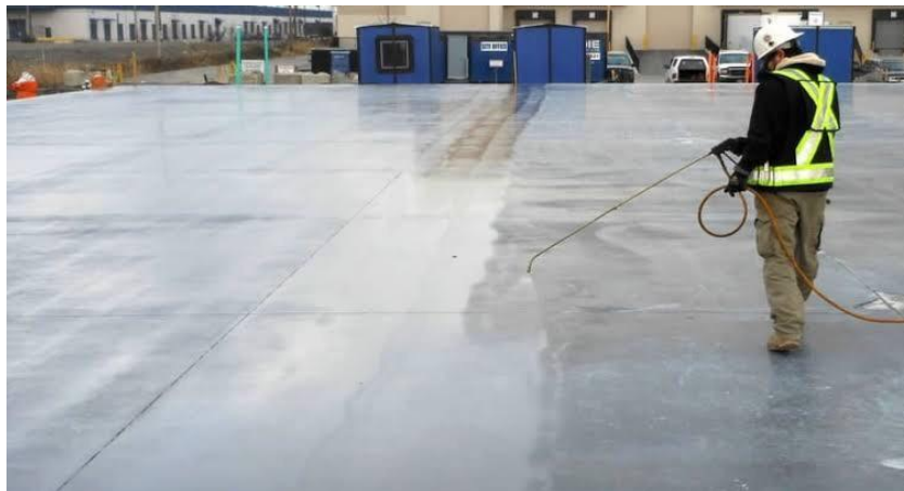
Figure 2-7 Fine water spray curing.
