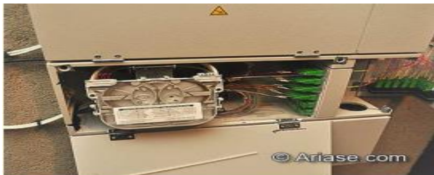
Figure 60: (2.39): Boite de raccordement immeuble.
