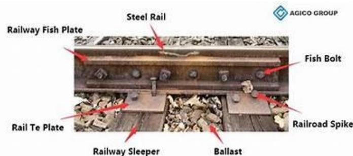
figure 2. 4: Components of a railway (AGICO group, 2017)
