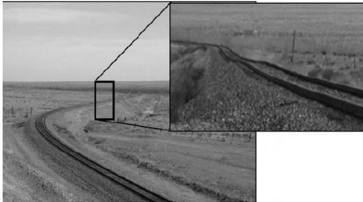
**figure 2. 27: Track settlement zone due to insufficient compaction of ballast.( Railway Geotechnics, Dingqing Li, James Hyslip, Ted Sussmann, Steven Chrismer)**
