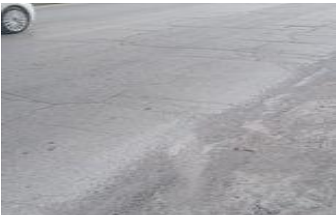
Figure II.15 faiçençage a maille large (degré01)
