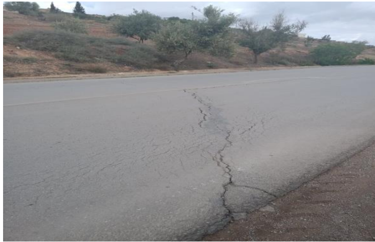
Figure II.14 fissures transversales
