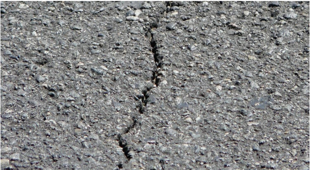
Figure II.6-fissure transversale- (Arbitusvinyl.com). [6]
