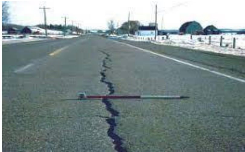
Figure II.7-Fissuration longitudinale- (bv.transport.gouv.qc.ca). [7]
