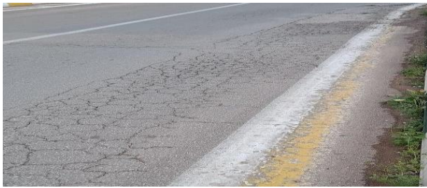
Figure II.16 faiçençage a maille Serrée ( degré 03 )
