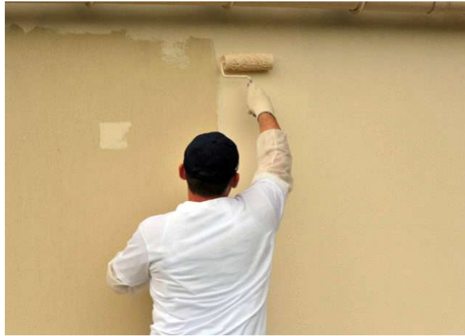
Figure 1.6: application de l'hydrofuge [Alain, 2015]
