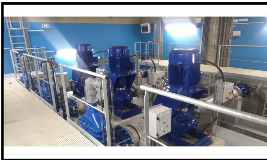
FigureIV.37. Station de surpression (XPAIR, 2013)
