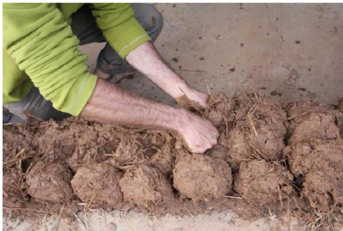
**Figure 1-9:** Construction en bauge.
