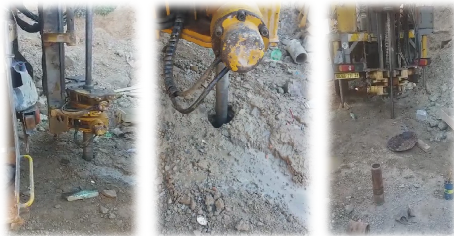
Figure (3.17): Essai de sondage carottier
