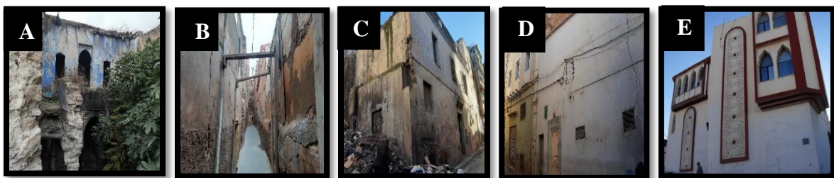
Figure 18: Etat de ruine Figure 19: Etat menace Figure 17: Etat médiocre Figure 16 : Etat moyen Figure 15: Bon état
