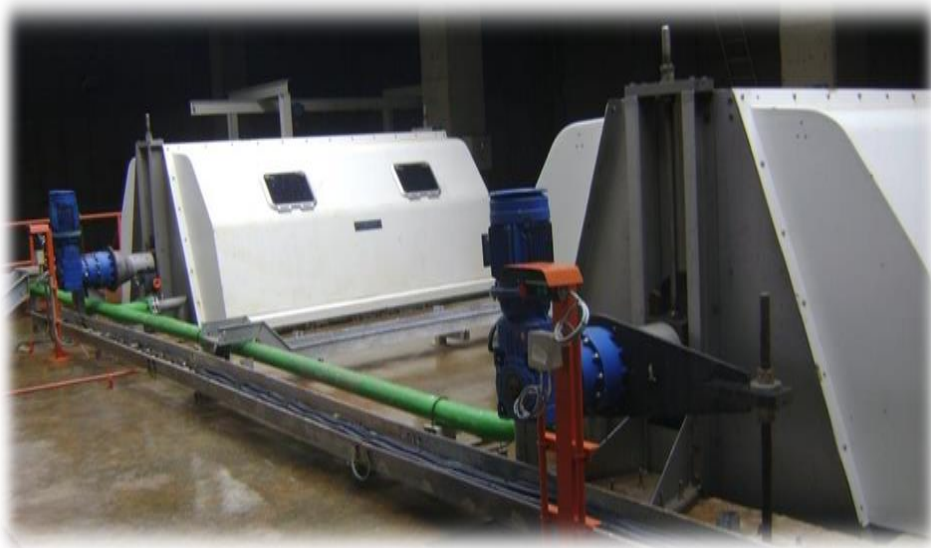
Figure 23: Filtres rotatifs
