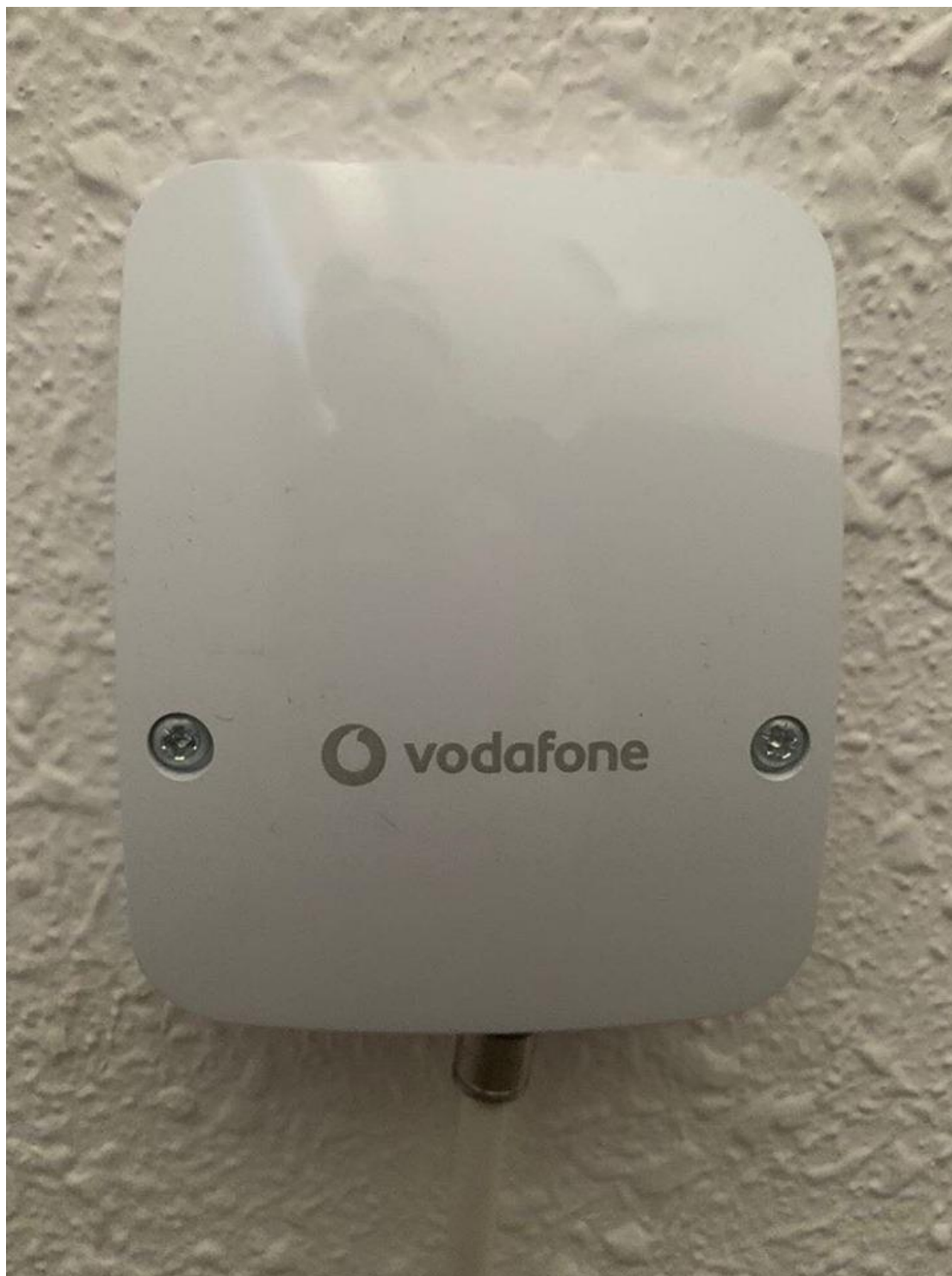
Figure II.5 : Prise Terminal Optique [30]
