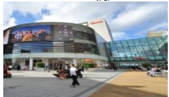
Figure1: 23 : Centre commercial Stratford source (www.gentside.cominsolitele-plus-grand-centre-commercial-d-039-europe-a-ouvert-a-londres_art27604.html).londres
