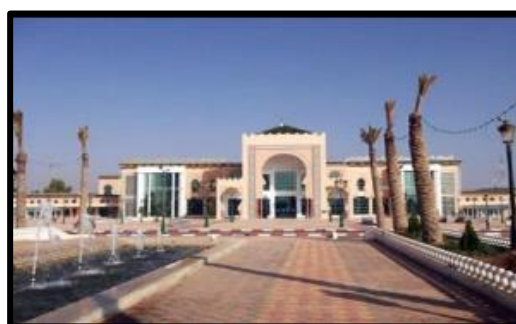
Figure 25: Aéroport Messali : source https://www.pinterest.com/pin/470485492
