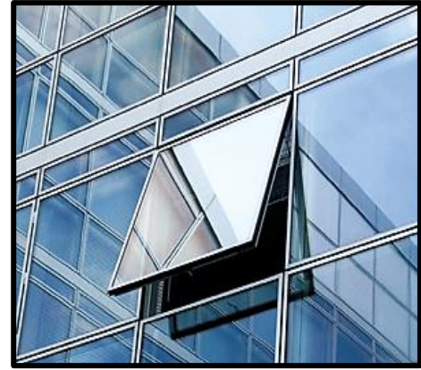
Figure 142: Mur rideaux VEC Source : https://www.riouglass.com/solutions/rglass-facade.html
