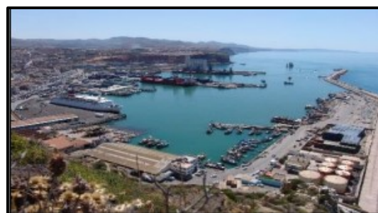
Figure21: Port de Ghazaouet
