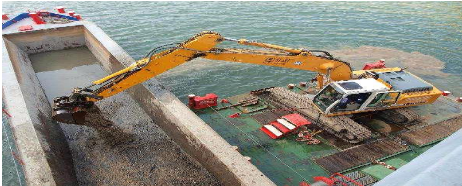
Figure 1.3 Dragage mécanique (BOUKEMMOUM N., NOUAOURIA A. (2019))
