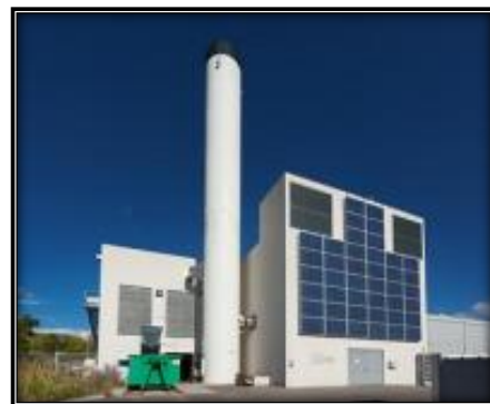
Figure 56: La chaufferie bois
