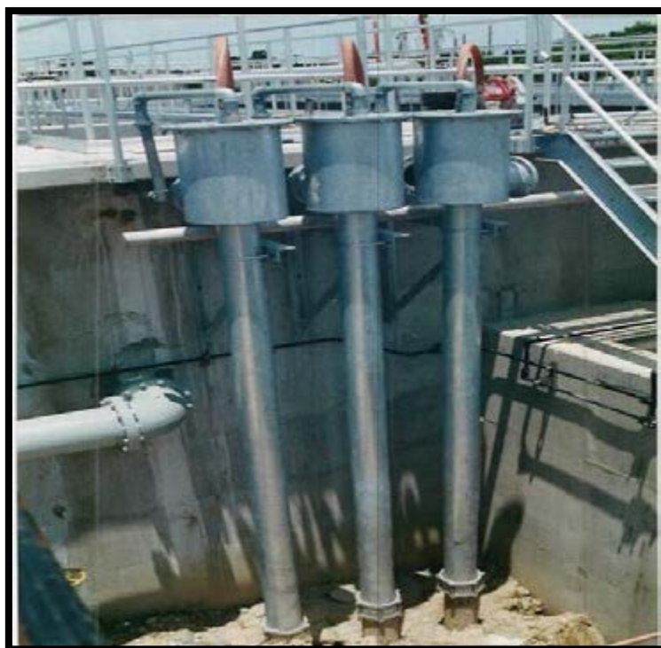
Figure IV.17 : Pompe Air-lift.
