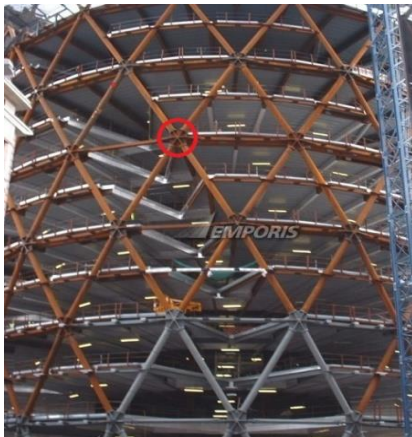
Figure 221 : Noeud de diagrid
