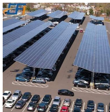
Figure : Eclairage solaire (parking).
