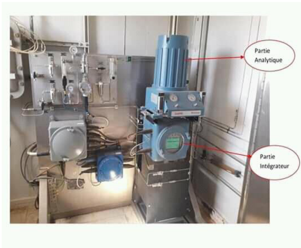
Figure I.13: Chromatographes Daniel Model GC700 [1].
