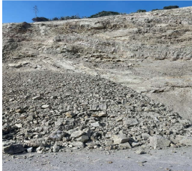
Figure 4.6 : Photographies de la section PK0+330-PK0-700
