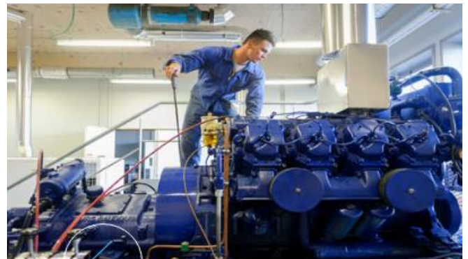
Figure 16: partie machine du bateau (Source : https://www.imq.qc.ca/techniques-de-genie-mecanique-de-marine )
