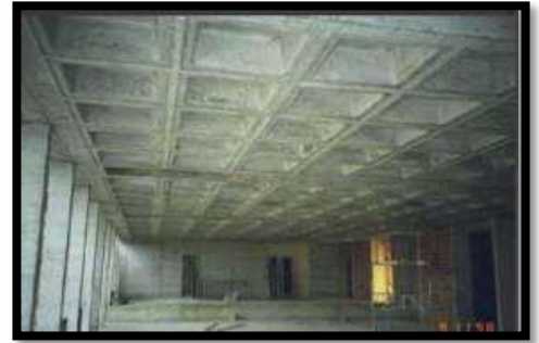
Figure 191: placher a caisson https://www.geoplastglobal.com/sites/default/files/catalogue_skydome_fr_0.pdf
