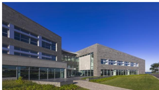
Figure 63: la façade sud
