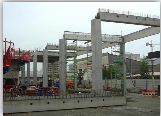
Figure 121: Structure poteau poutre
