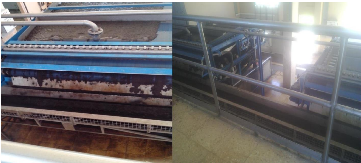
Figure II.19. Bande presseuse (Terga)
