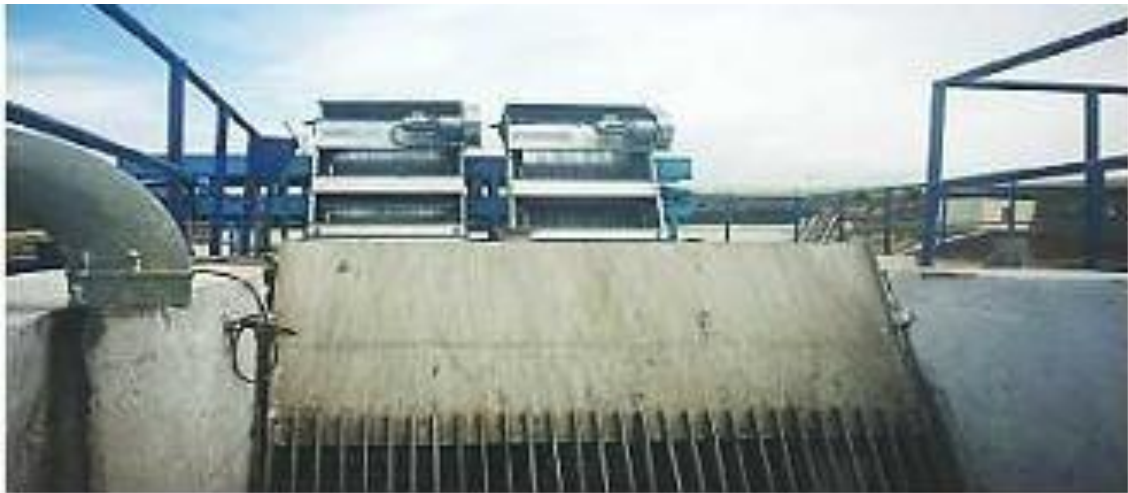
Figure II.21. Grille grossière manuelle (Ain El Houtz)
