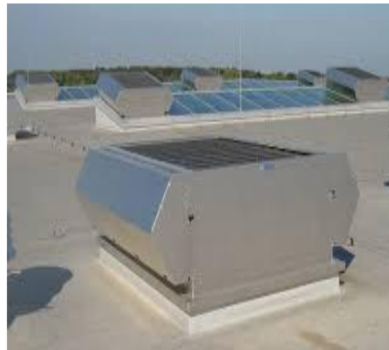
Figure I.14.:Bouches des extractions
