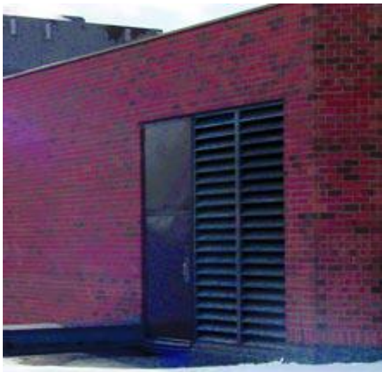
Figure I.14.:Bouches des extractions
