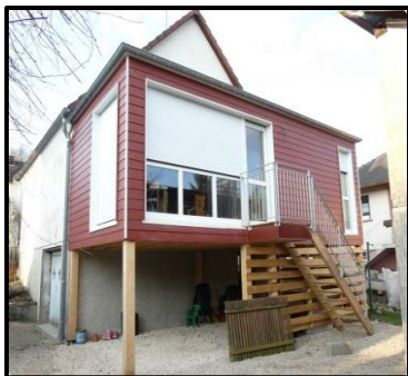
Figure 18: extension en conteneur
