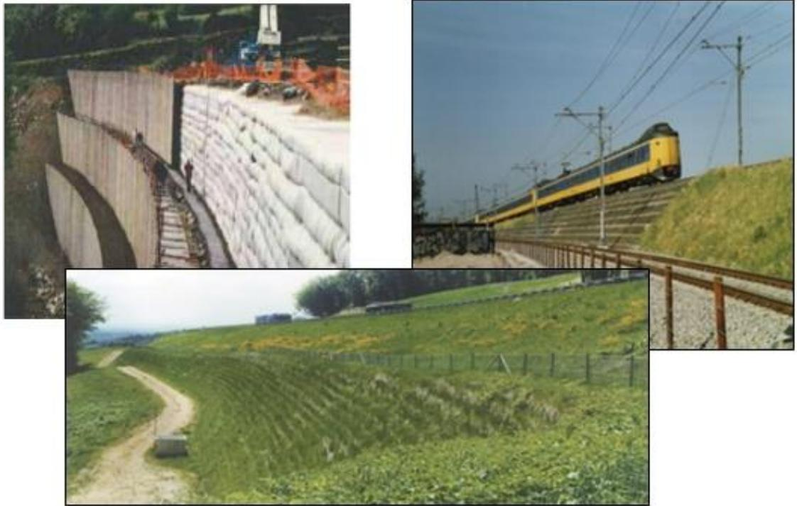
**Figure 3-9** Parement face enveloppée
