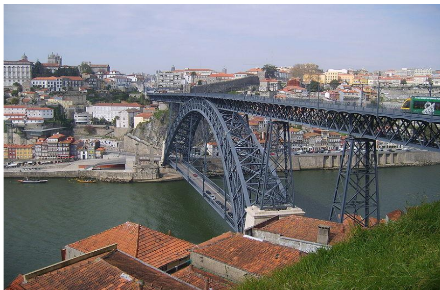
Photo.2.5 Pont Dom Luis I.(5)
