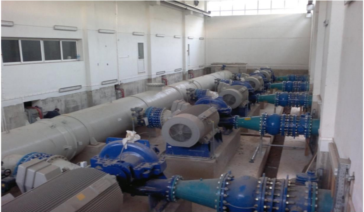
Photo II.4 Installation des pompes HSP1 [27]
