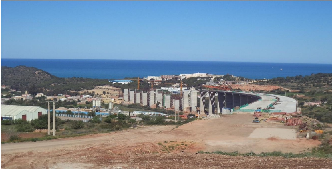
Figure 24: Photo du site
