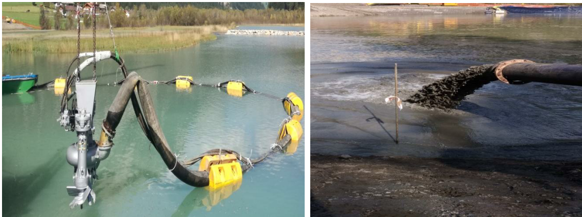
Photo I.2: Le curage hydraulique [11]
