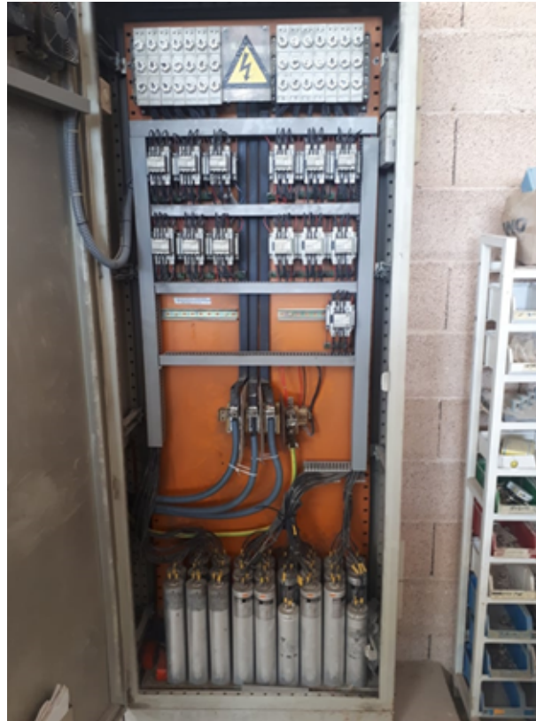
FIGURE III.8 – Armoire de compensation en gradin
