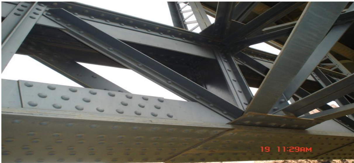
Figure 1.16.2.1 Le rivetage.
