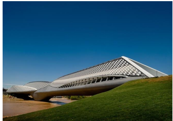
Figure 21 : Vue générale su pavillon pont de Saragosse. Source: http://buildipedia.com/images/masterformat/aec/2013.03.18_zaha/images/Fernando%20Guerra/1199_FG_094.jpg
