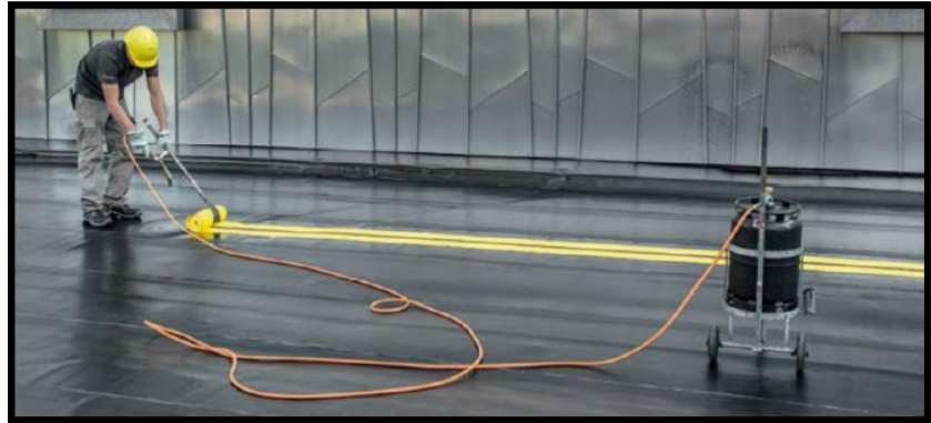
Figure 158: Technique de couvre joint
