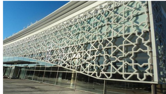
Figure 147. Exemple de la double peau (source : https://www.ductal.com/sites/ductal/files/atoms/files/ductal_solutions_ndeg15_fr.pdf )
