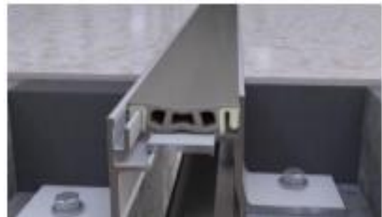
Figure 130:couvre joint
