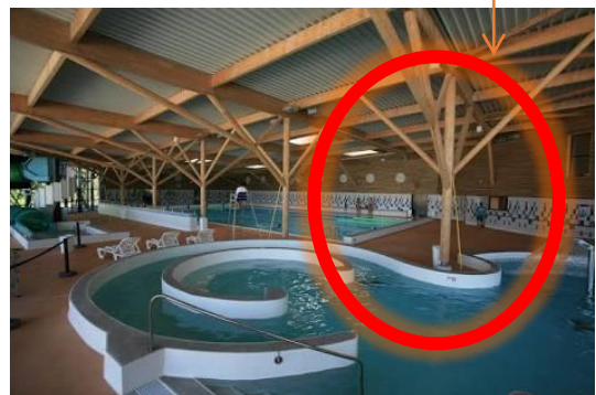
Figure 90:la structure en bois
