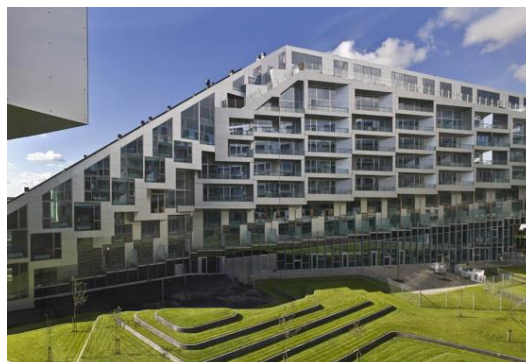
Figure 4-21: façade nord source:
