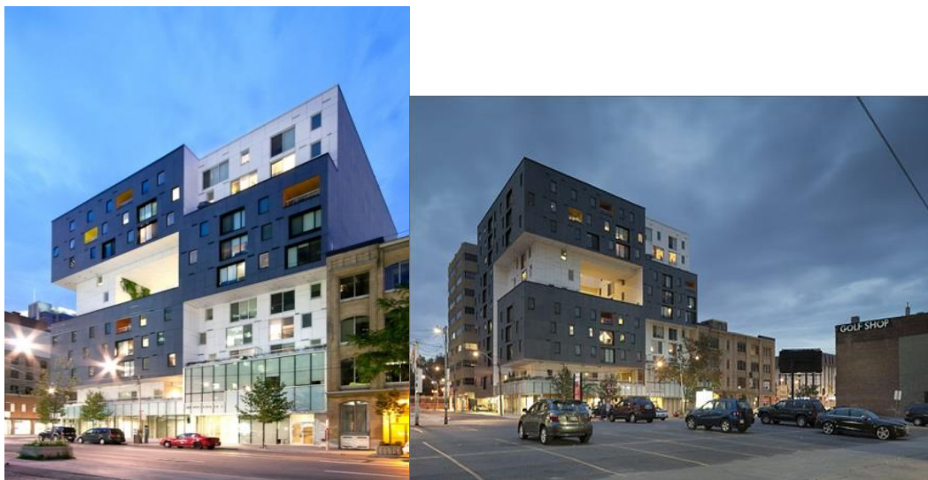
Figure 4-31: situation Vues panoramiquesdu la projet source: https://translate.google.dz/translate?hl=fr&sl=en&u=https://www.archdaily.com/85762/60-richmond-housing-cooperative-teeple-architects&prev=search
