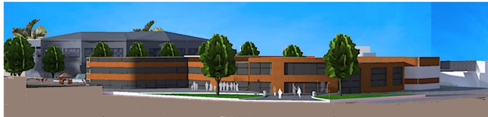
Façade principale de centre commercial
