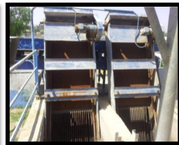
Figure 32: Grille de by-pass Figure 33: Grille grossière Figure 34: Grille fine
