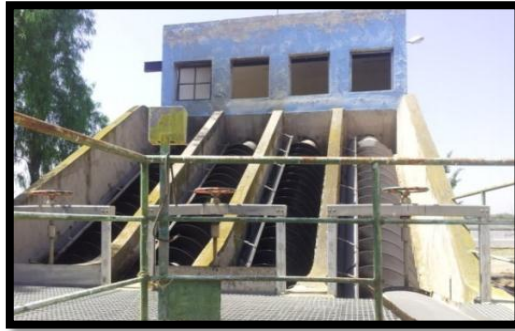
Figure 36 : vis de relevage
