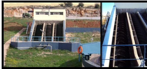
Figure 21: Vis de recirculation
