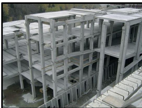
**Figure 89.** Structure poteaux-poutres
