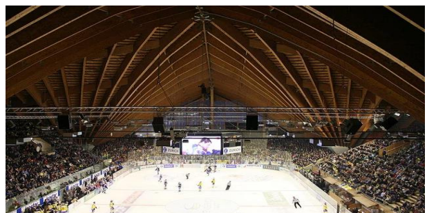
Figure 10 Vaillant Arena Switzerland
