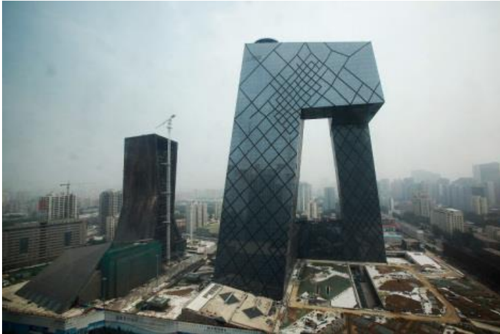
Figure 110 : Tour CCTV, Chine
