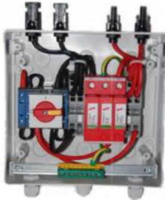
**Figure(III.24) :Protection courant continu[17]**
