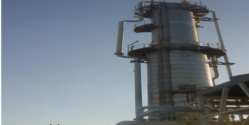
Figure I-1 : Colonne de distillation
